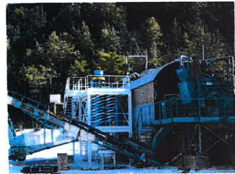
G.S.I. Bonnevault. Installation des "spires" 22-09-2002
